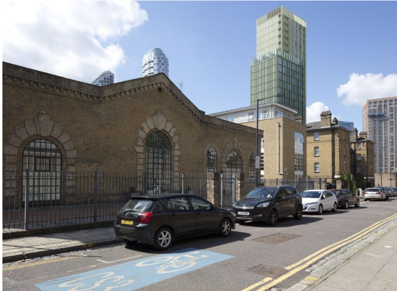
Figure 15: View 2 (Naval Row CA & Listed Pumping House)
