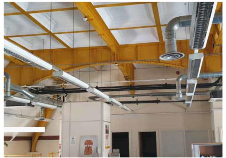
Figure 5: View of roof structure to existing office building
