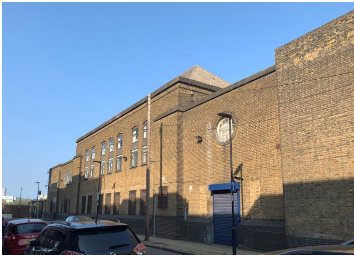
Figure 4: View of existing office building
