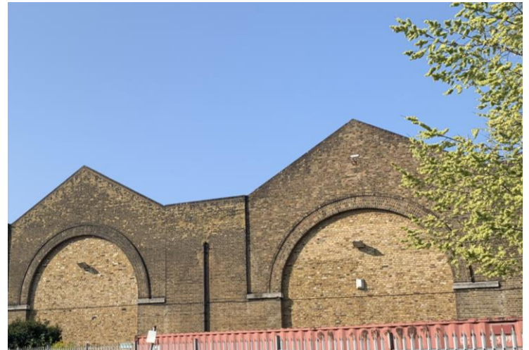
Figure 3: View of tram shed arches and gable ends
