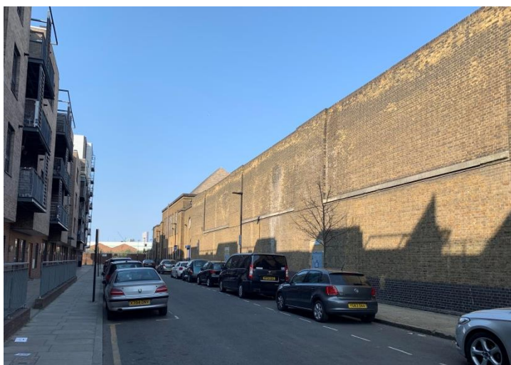
Figure 6: View of 9m high boundary wall
